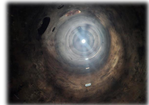
Stove shell after demolition of old refractories
